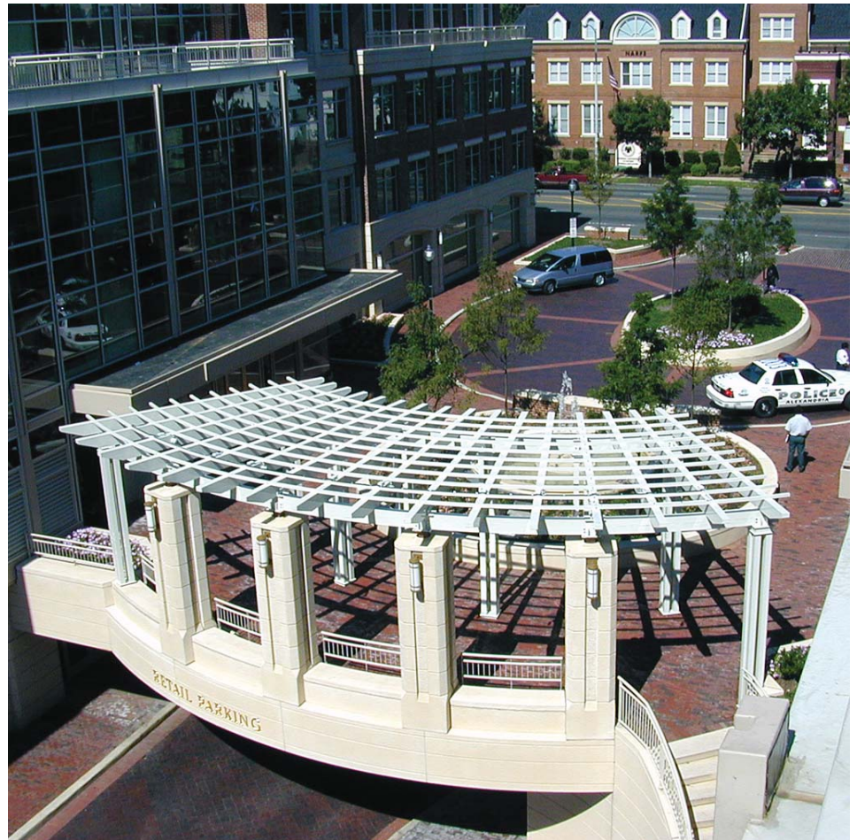
View of North Washington Street Entrance and Pergola
