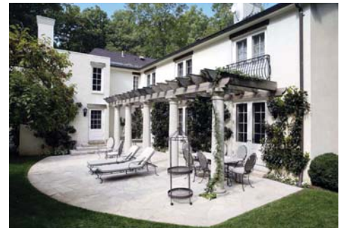
View of limestone terrace and cedar pergola after construction
