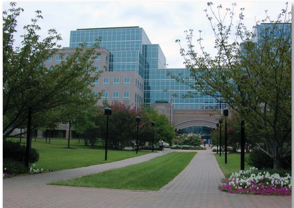
View of entrance walkway
