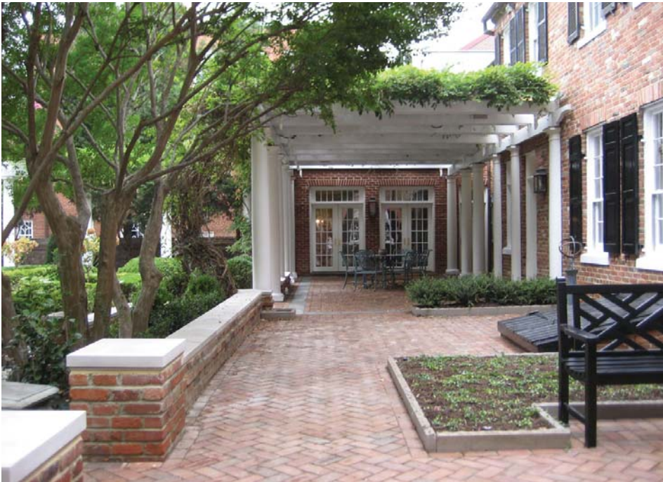
View of modified patio, brick paving has been reset in mortar with bluestone accents, planter beds with limestone edging and updated brick walls with limestone coping
