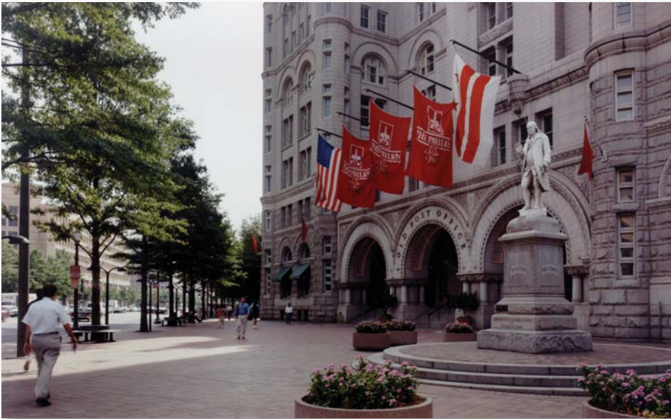
View of main entrance to the Old Post Office building
